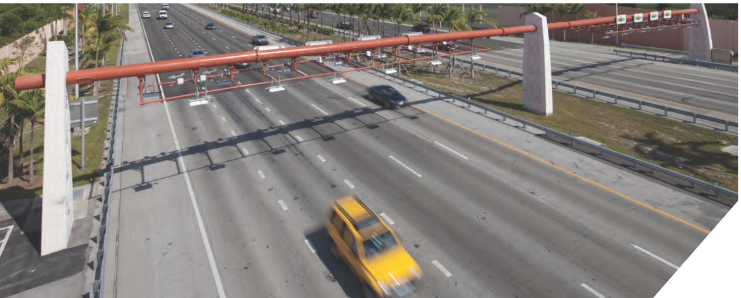
SR 874 Toll Gantry, ORT, AET
